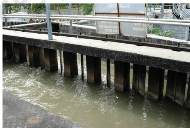
Fig. 18.4 Grit and sand removal tank
