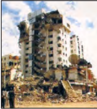
Fig. 3.3a: Destruction caused by an Earthquake in Gujarat
