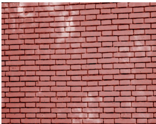
(a) Brick wall
