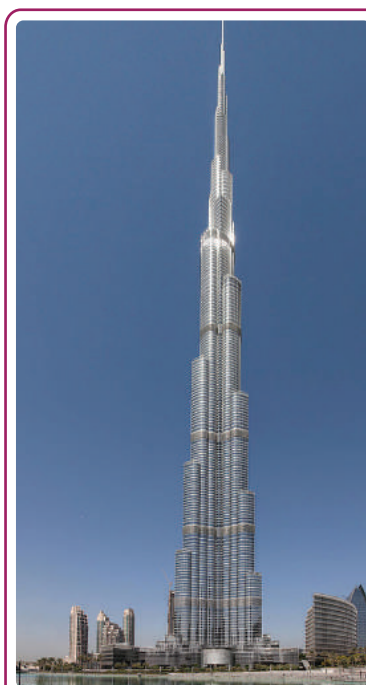
Fig. 2.1 , Burj Khalifa, an 828 m tall building located in Dubai; Image by King of Hearts via Wikipedia
