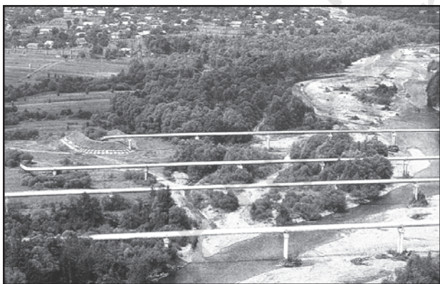
Fig. 8.17: Pipelines transporting natural gas in Ukraine
