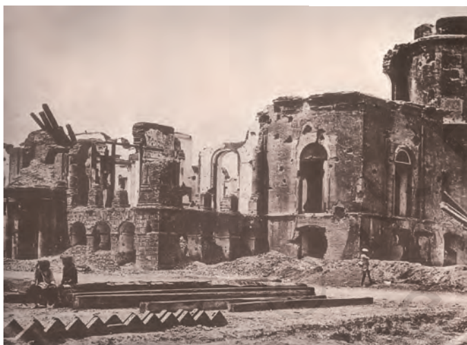
Fig. 17 – Ruins of the Residency in Lucknow
