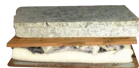
Figure 56.4 Sunmica sheet over wet paste and block of stone over it
