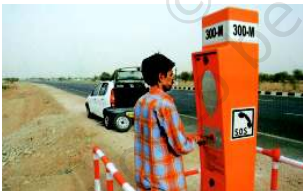
Fig.7.10 : Emergency call box on NH-8
