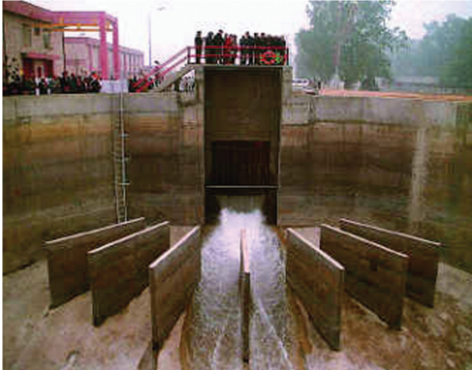
Fig. 18.10 : Water treatment plant
