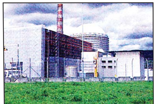
Fig. 3.18 : Nuclear power station , Kalpakkam
