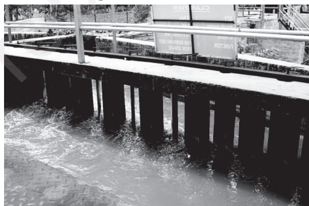
Fig. 18.4 Grit and sand removal tank
