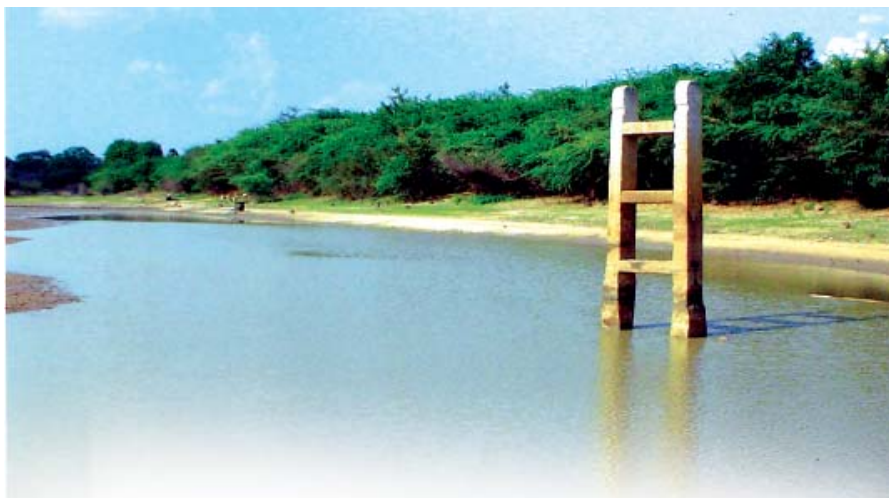
Fig. 5 A ninth century sluice-gate in Tamil Nadu. It regulated the outflow of water from a tank into the channels that irrigated the fields.
