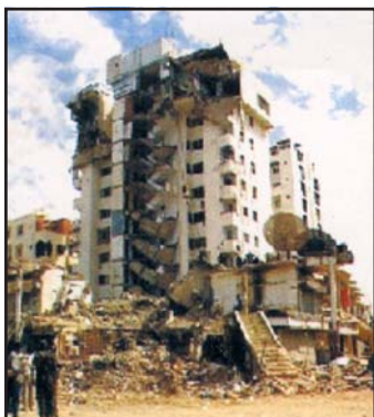
Fig. 3.3a: Destruction caused by an Earthquake in Gujarat
