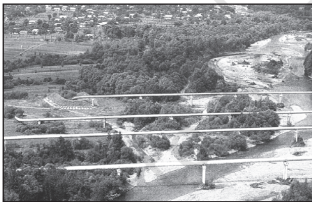
Fig. 8.17: Pipelines transporting natural gas in Ukraine
