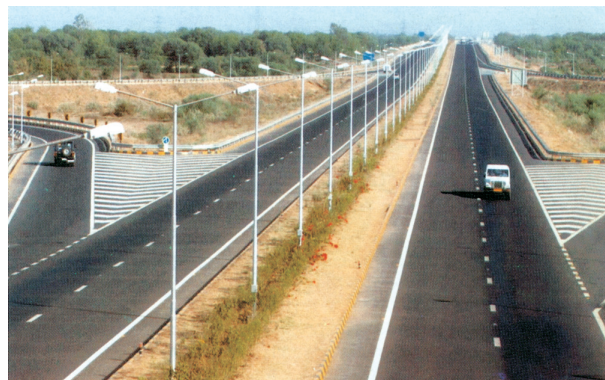
Fig.7.2: Ahmedabad- Vadodara Expressway
