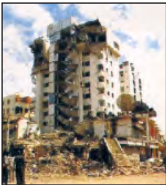
Fig. 3.3a: Destruction caused by an Earthquake in Gujarat
