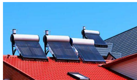
Many housing societies have started installing solar panels on the top of their house for lightening lobbies and heating water.
