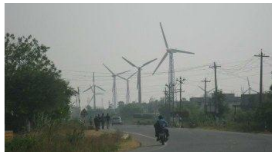
The largest wind farm in India is situated from Nagarcoil to Madurai in the state of Tamil Nadu
