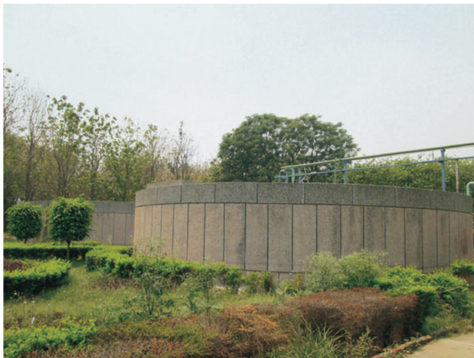
Fig.11.3. Effluent treatment plant
