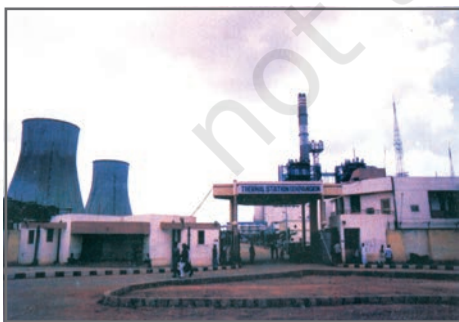
Fig 3.10: A view of a Thermal Power Station
